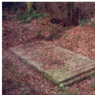
4 Settlement tanks near stream
